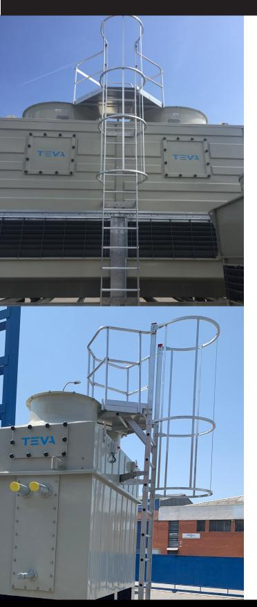
New optional: Ladder with ring protection and inspection platform. They are designed to fit on any of our axial series: TVAE, TVAES, TVAP, TGA, RVA, RVAS, RMA, CVA, CVAS and CMA.
